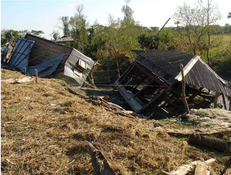
Small shops, businesses, market areas, damaged along the road side.
